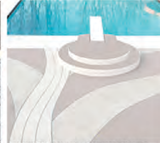
COLORED CONCRETE WITH PATTERN AT POOL DECK
