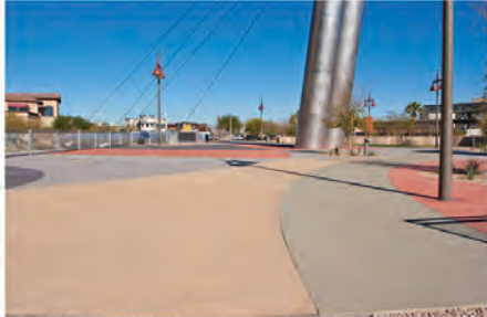
INTEGRAL COLORED CONCRETE
