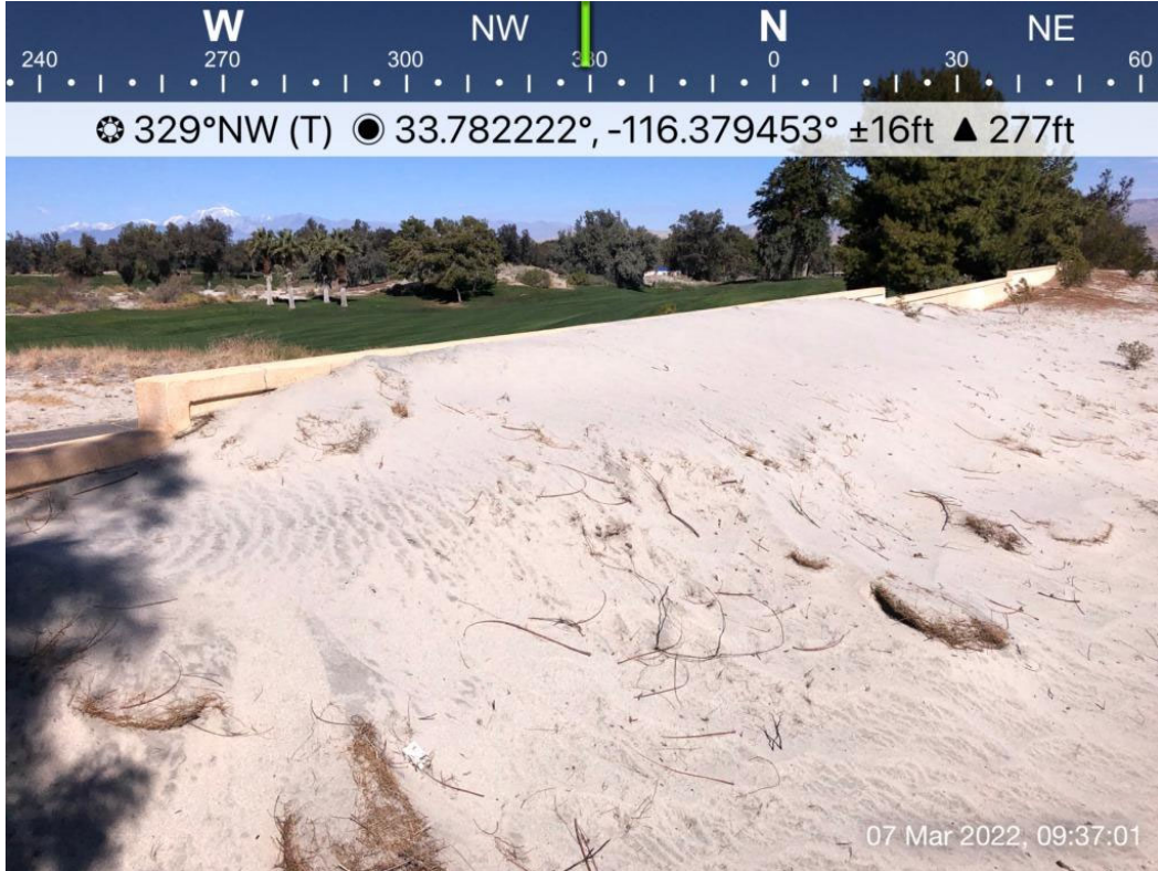
Photo 5. Dune / blow-sand from site overtopping the golf course wall on west boundary.
