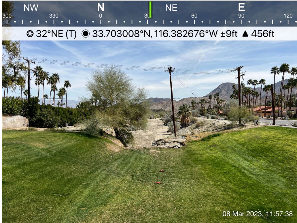
Photo 3. Looking east, east of Heliotrope Drive showing the transition from turf swale to sandy wash.
