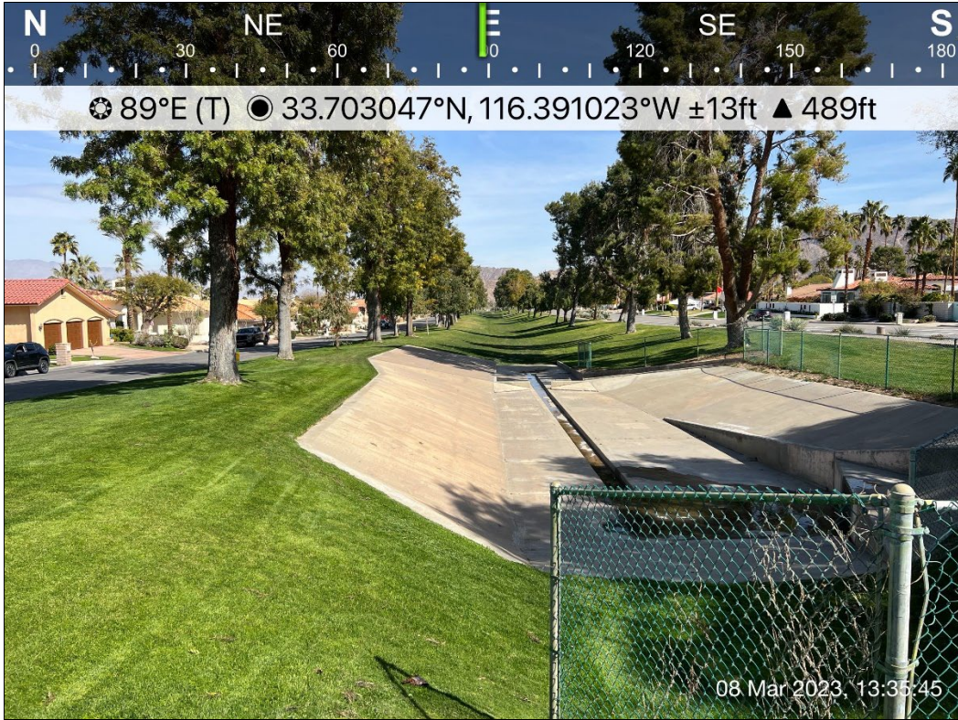
Photo 1. Looking east from Alamo Drive showing the grass swale and concrete facilities for nuisance waters.
